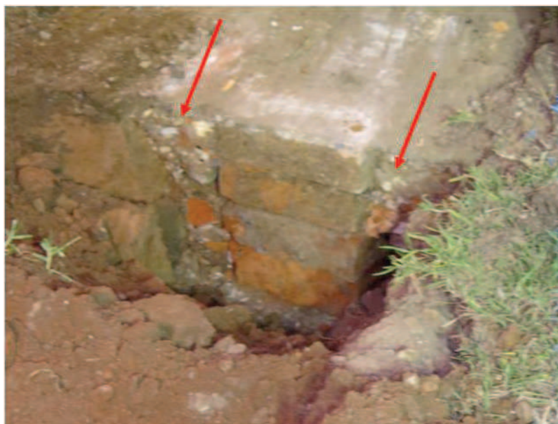
Figure 3.12: The sandstock brick shop footing found in the northern pit on the corner of Harris and George Streets. Construction fill is arrowed red. Taken during night monitoring. C&L 2013.
